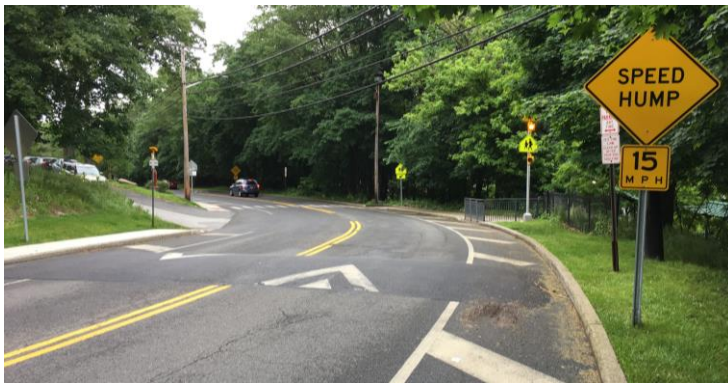
ONE OF TWO SPEED HUMPS USED TO CREATE A TRAFFIC CALMING SLOW ZONE AROUND THE CROSSWALK TO THE TOP OF THE SPRINGHURST ELEMENTARY SCHOOL STAIRWAY
